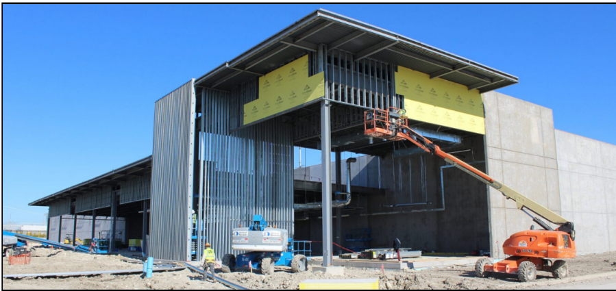
Tilt-up construction with steel frame front offices will reduce cost
